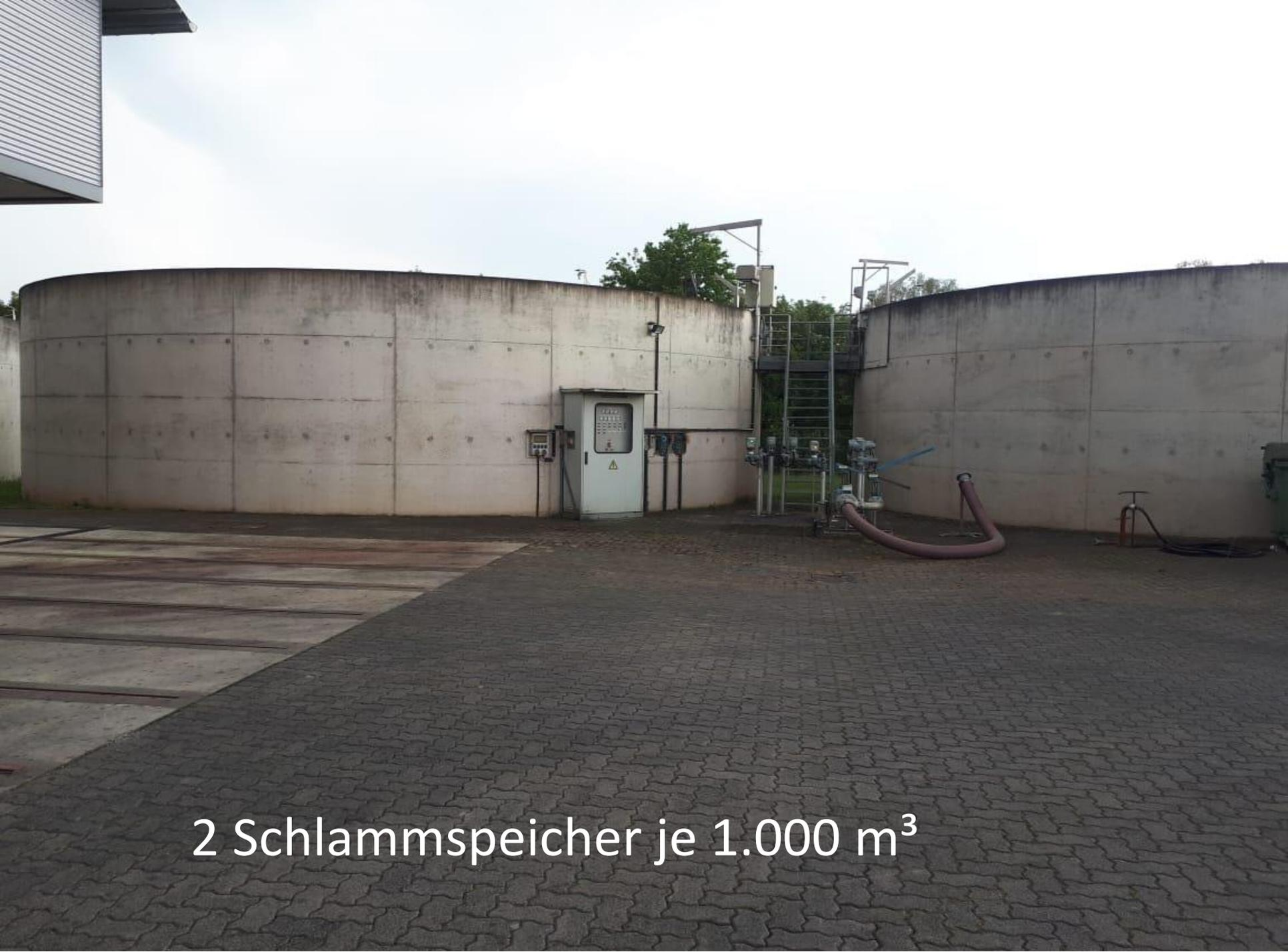
The image shows two large, cylindrical concrete tanks used for sludge storage. The tanks are situated outdoors on a paved area. Between the tanks, there is a white electrical control cabinet with a warning symbol, a staircase, and various pipes and valves. A red hose is coiled on the ground near the tanks. The sky is overcast.
